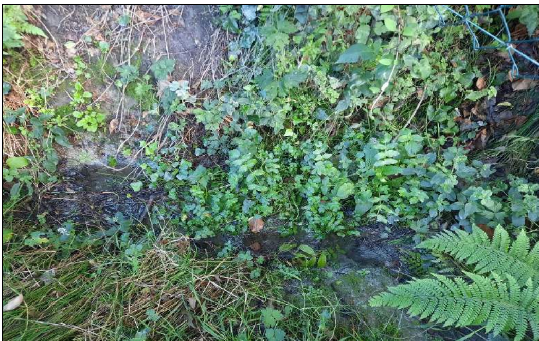
Figure 5-8 Drainage ditch on southern Site boundary.
