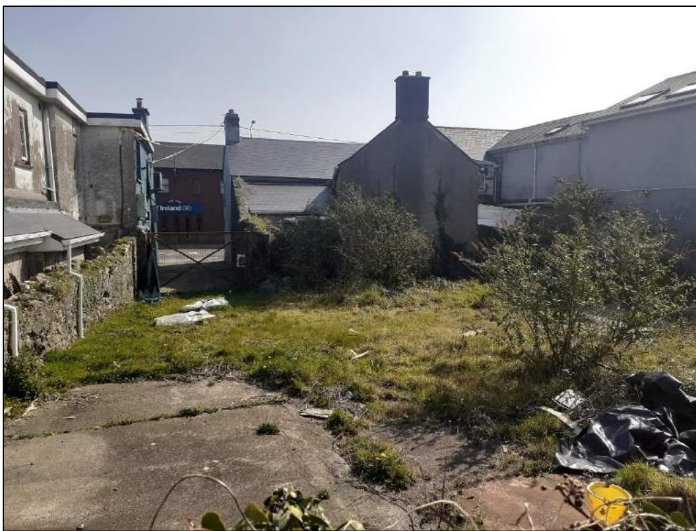
Figure 5-3 Existing buildings and yard along proposed access route to Carrigaline main street.
